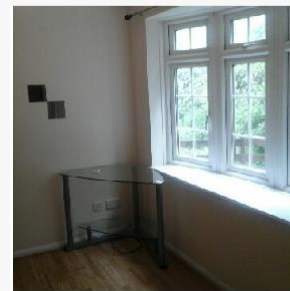
No cracked glass on the windows and was in clean condition 29/11/2016 10:22 (GMT)
